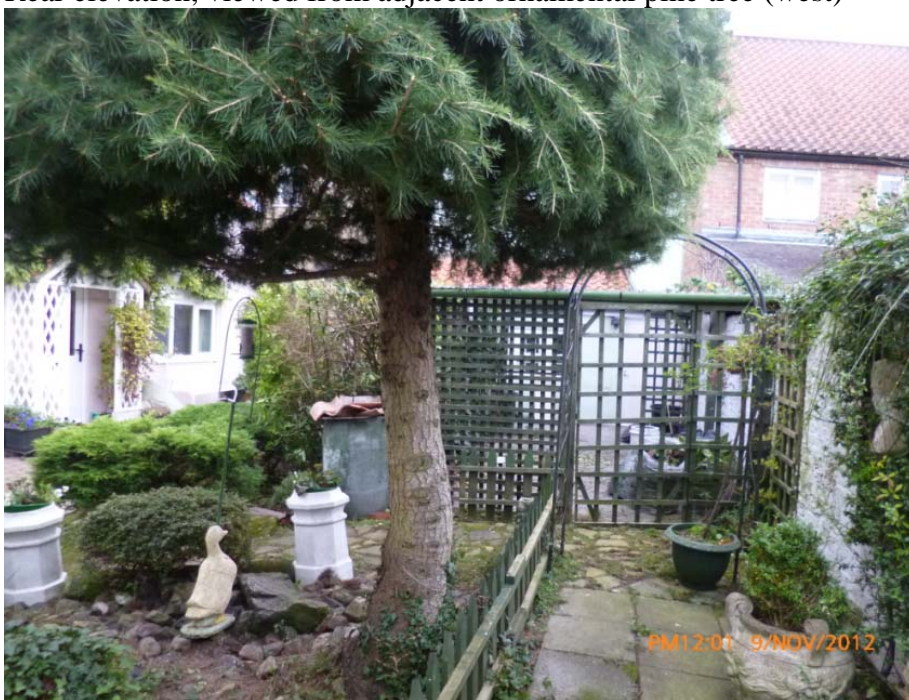
Rear elevation, viewed from adjacent ornamental pine tree (west)
